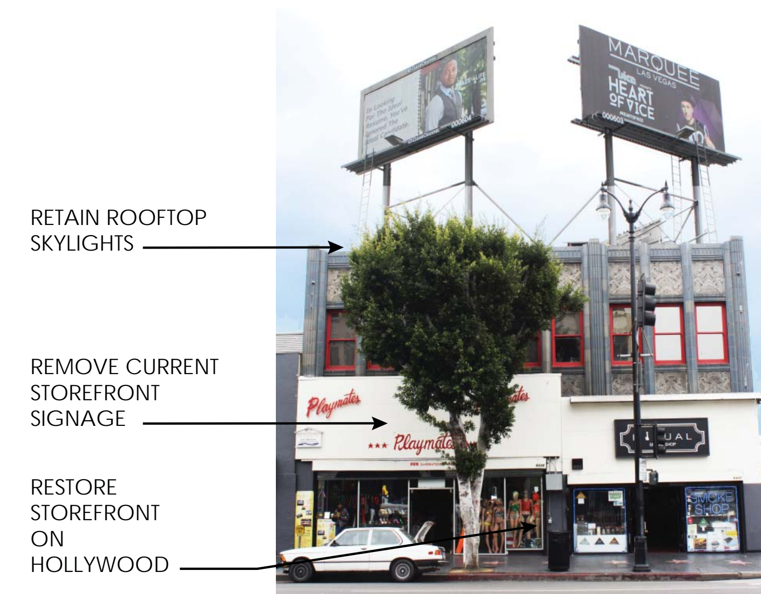
PHOTO ALONG HOLLYWOOD BLVD. GMPA | 2016
